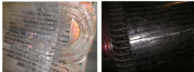
Figure 1. Contact of the rotor with the stator of the induction motor due to the presence of static eccentricity
